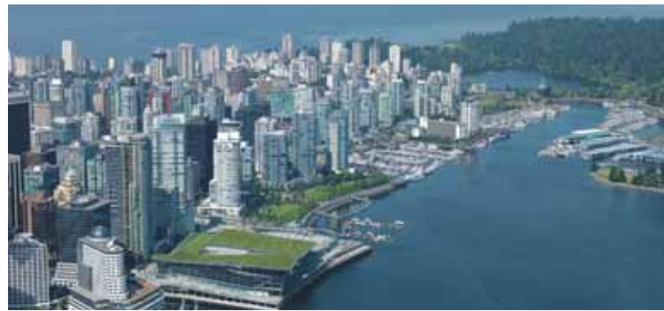
GOING GREEN. The roof of the Vancouver Convention Centre is a six acre 'living' roof
